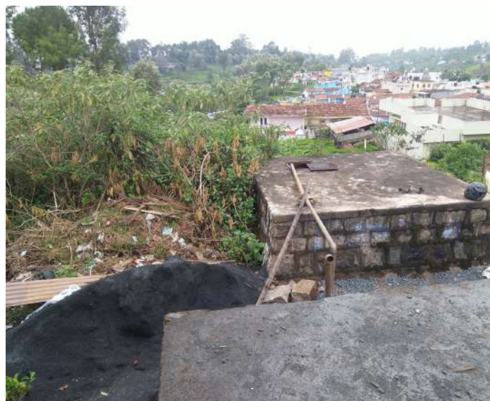
The repair of a ground-level reservoir is conducted in Horosholai.
