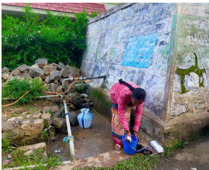
As part of our Water and Sanitation projects, our team regularly monitors water quality across several regions.
